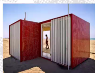
5G Module (Technical Room)
