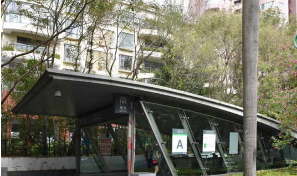
The Metro Entrance of Qiaocheng East Station @ Shi Yin
