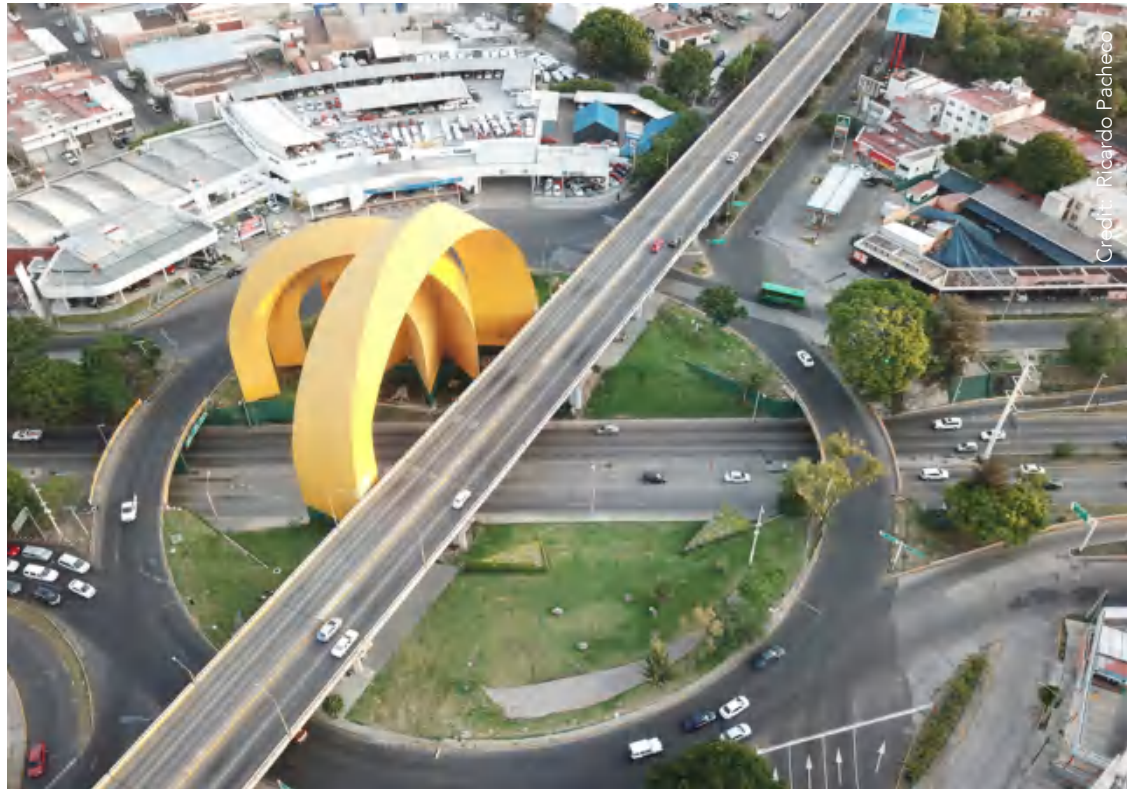
Aerial view of the Andares and the Puerta de Hierro neighbourhoods. Guadalajara, Jalisco, Mexico.
