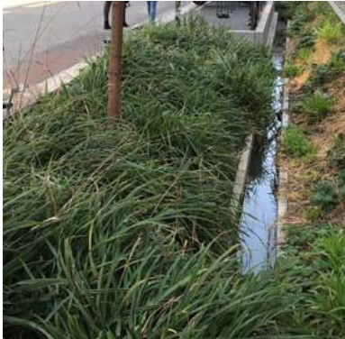
SYSTEM OF TRENCHES FOR RAINWATER MANAGEMENT
