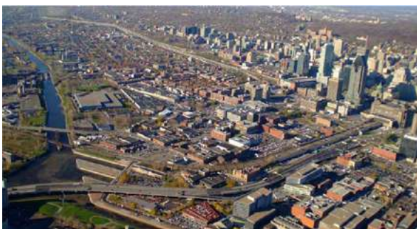
AERIAL VIEW OF GRIFFINTOWN IN 2013
