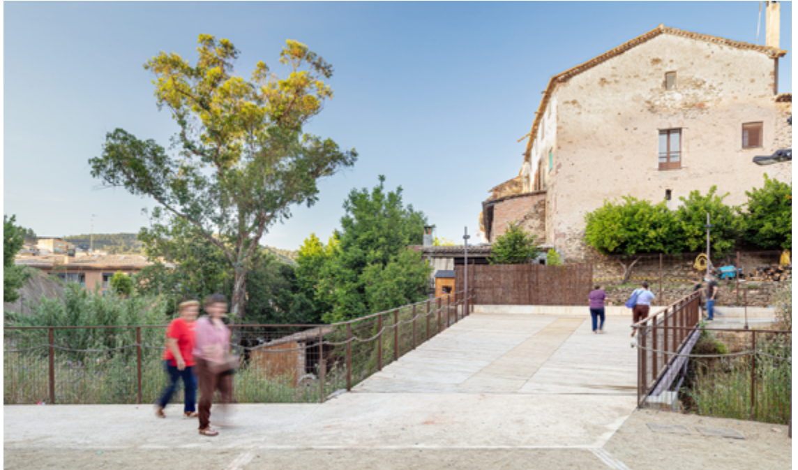
Renovation of Font del Rector. © Adrià Goula
