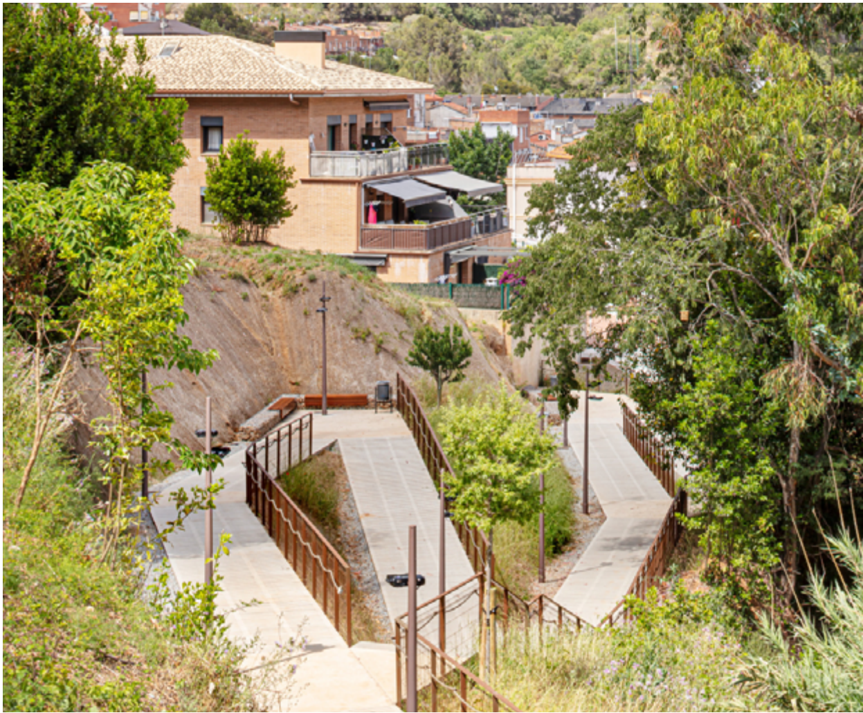
Renovation of Font del Rector. © Adrià Goula
